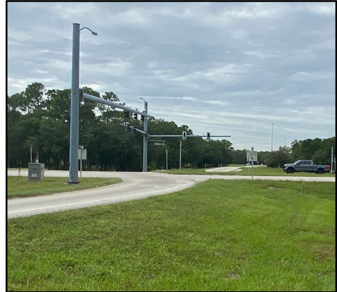
I-95 southbound off-ramp at the intersection of Midway Road (pre-construction)
