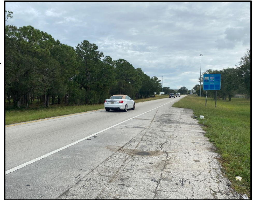
Northbound I-95 off-ramp at Midway Road (pre-construction)
