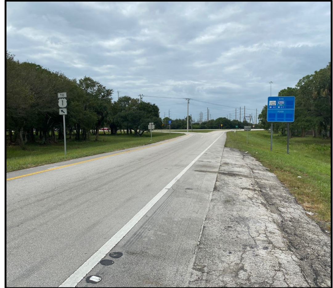
I-95 southbound off-ramp to Midway Road (pre-construction)
