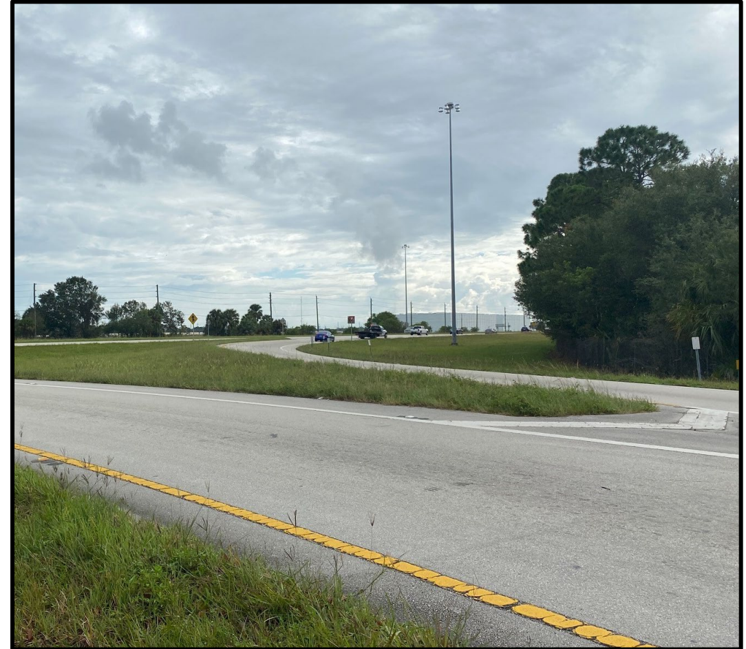
I-95 northbound off-ramp to Midway Road (pre-construction)
